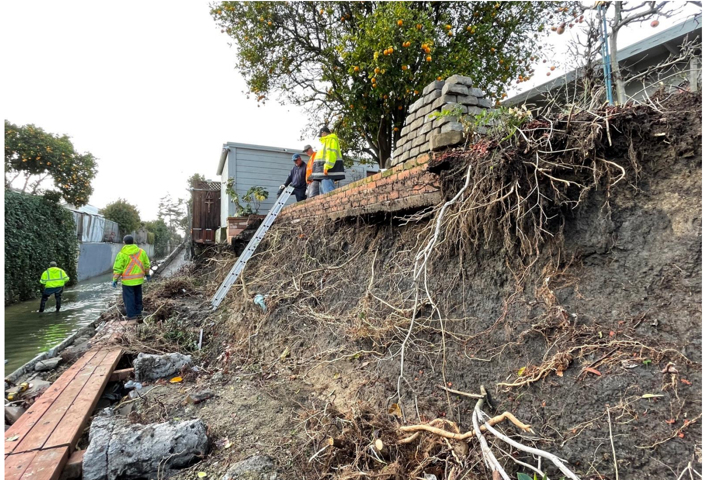
Estudillo Canal in San Leandro after early January 2023 storms
